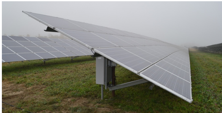
Figure 8 - Ground Mount System
